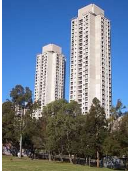
Plate 3. South Korea Tower block apartment (typical) Source: Internet (April 25, 2023)
